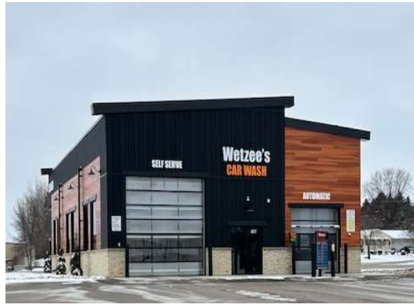
Wetzee's Car Wash (Ash Street NE)
